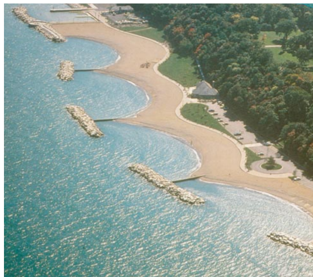
Breakwaters for captive beaches at Lake Forest, Illinois
