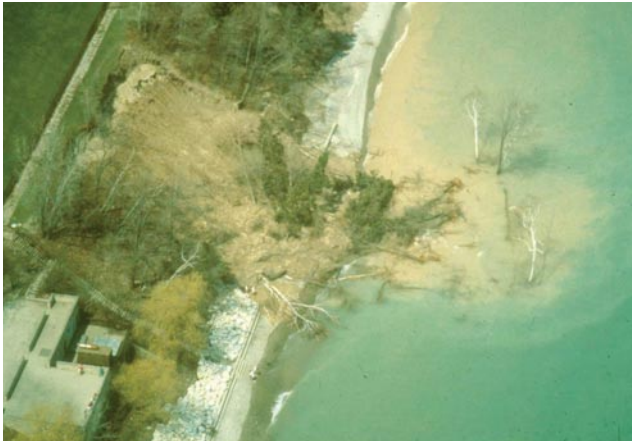
Bluff failure at Klode Park, Lake Michigan
